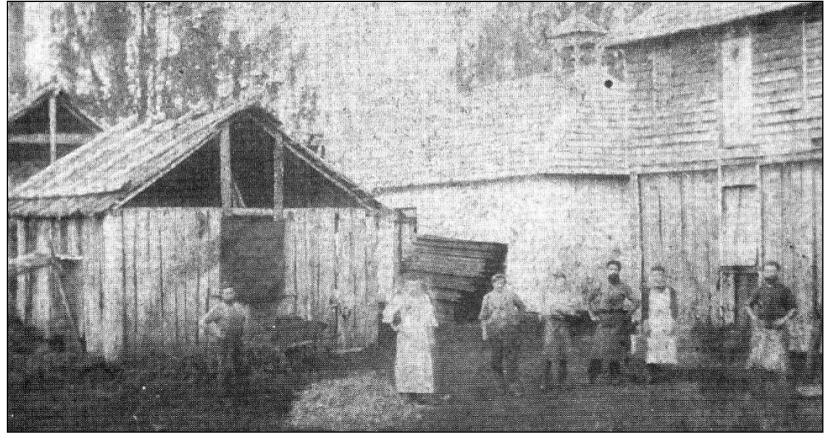
Figure 14 Photograph of the Tannery, Broughton Creek, c.1875 (In Mabbutt nd:6)
