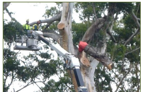
Figure 20 Removal of a hollow canopy branch, stopped at both ends to contain any potential residents for later release
