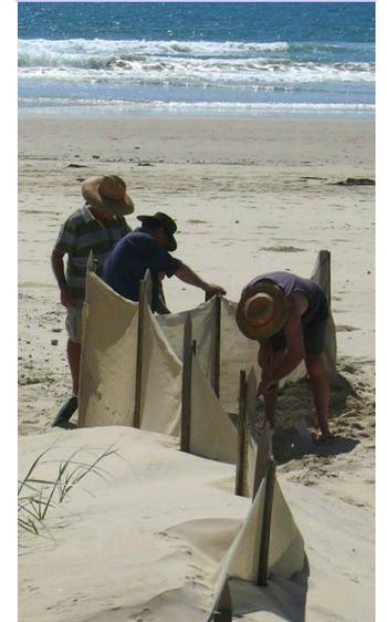
Construction of sand trap to prevent wind erosion and to enable Lake Cakora berm to rebuild
