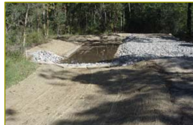
August 2009: Stilling Basin before planting out
