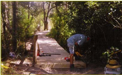
2005: 9th Bridge under construction.
