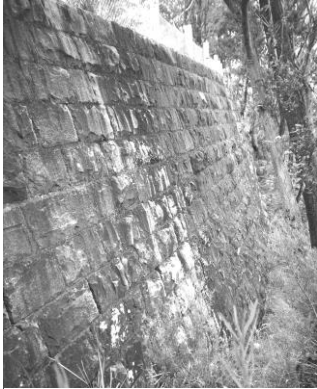
Loop Road Supporting Wall
