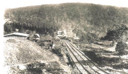
Double Light Rail to Crusher
