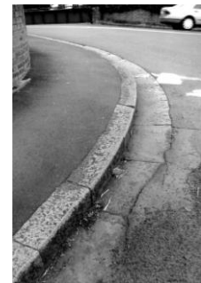
Kerb and Gutter
