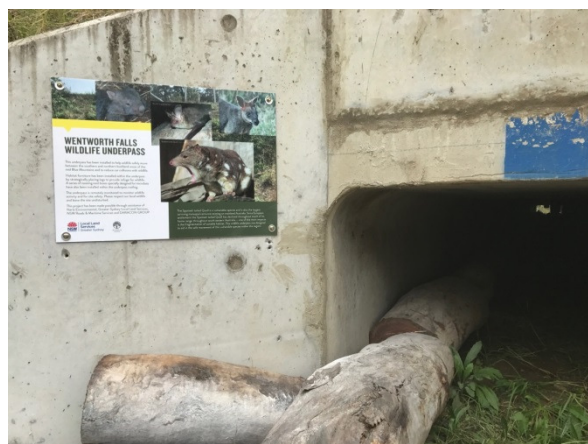
Wentworth Falls wildlife underpass
