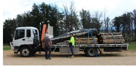
Delivery of geotech material and hardwood pins this week.
