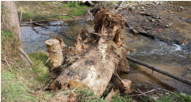
Rootball in situ with cable securing it to embedded posts
