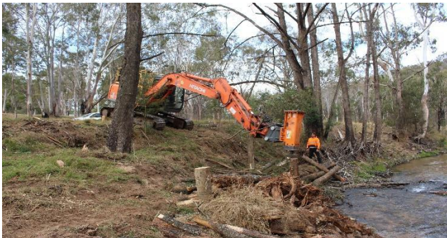
Hammering posts into bank stabilization structure
