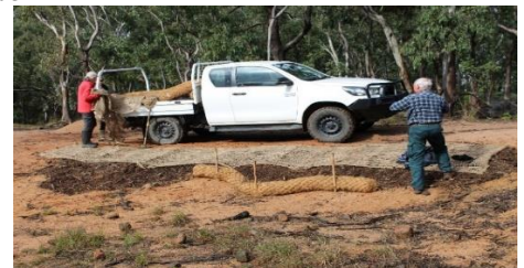
Coir log, jute matting & mulch demonstration
