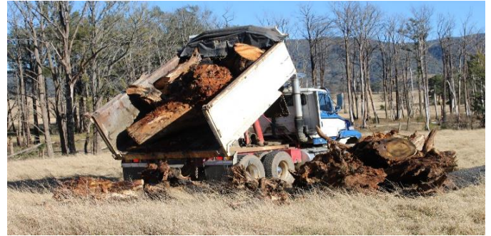
Rootball delivery to stockpile. Rootballs will be installed at various sites to minimize swirling and erosion. Strategic rootball placement reduces the energy of the flow.
