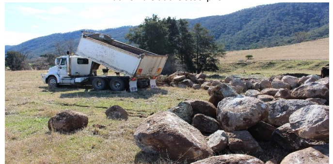
100 tonne of rock delivered to site 9
