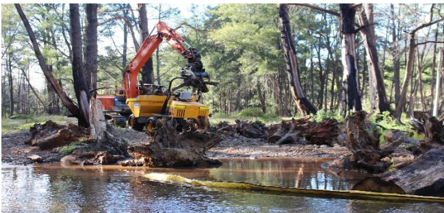
Reopening of the original channel, diverting flows and positioning rootballs to reduce impacts on severely eroded bank pictured below.
