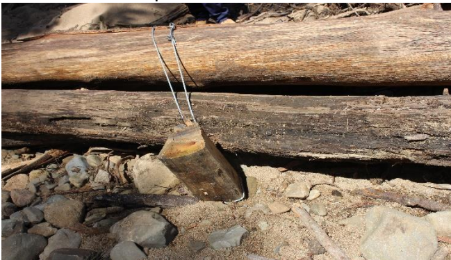
Technique of log pinning in order to provide stability & erosion control
