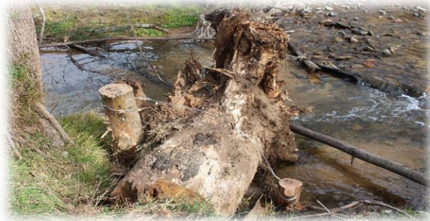
Rootball in situ with cable securing it to embedded posts
