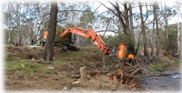
Hammering posts into bank stabilization structure
