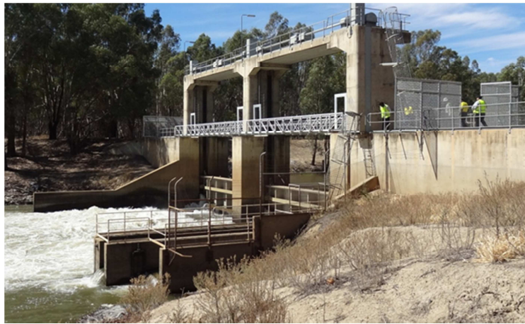
Image of the existing Yanco Regulator
