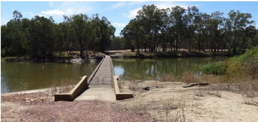
Image of the existing Yanco Weir
