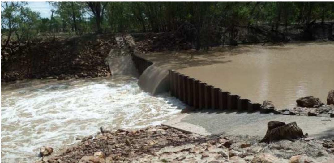
**Figure 3-3: Sheet Pile Weir (Donnegri Creek, Narran River, South west Queensland)**
