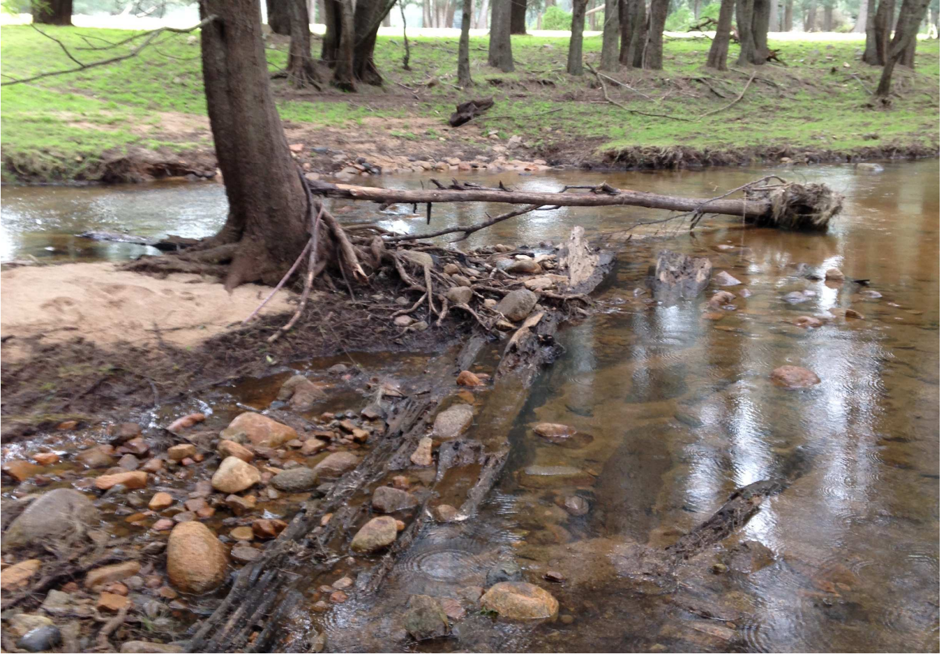
Figure 4: Log sill at site 10, in need of replacement of upper log/ potential upgrade.
