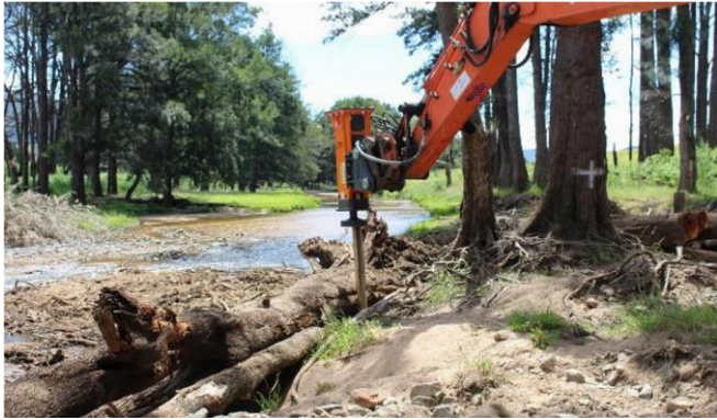
Hammering anchor points to cable tie logs in position.
