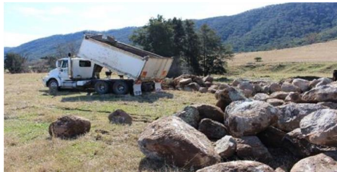
Delivery of rocks to site.
