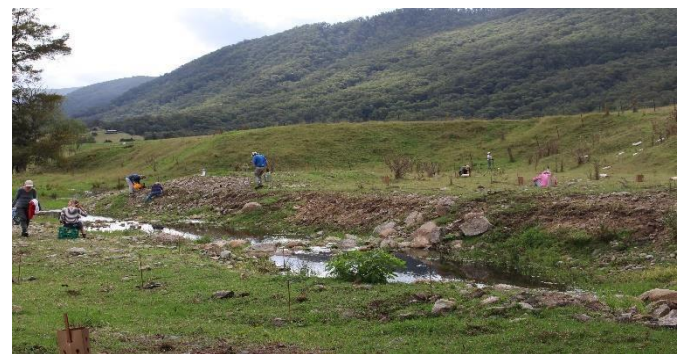
Planting Day 2 nd April 2023 – volunteers revegetating remediated site.
