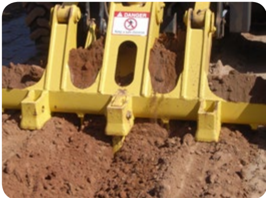
Final pass at full depth, producing a deep, friable planting bed suitable for seeds and seedlings. Note the scarifying bar is only approximately 0.5m wide. Try and avoid unnecessarily wide cultivation as it will reduce the effectiveness of the water harvesting.
